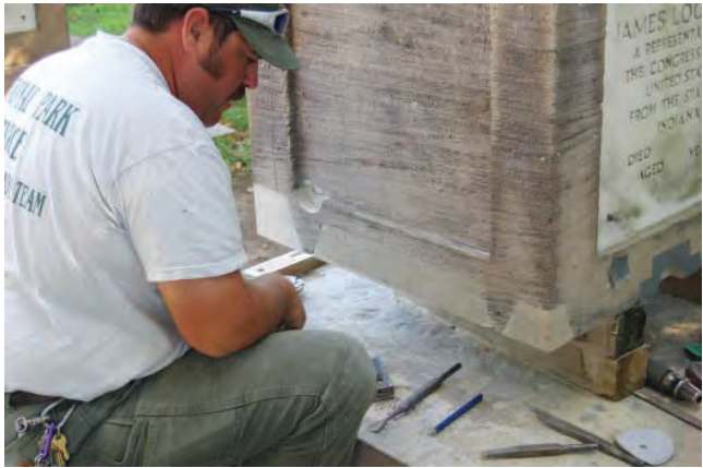
Figure 16. A professional mason works to insert a new piece of stone. Often referred to as a “dutchman”, this repair technique requires replacing the deteriorated stone section with a new finished piece of the same size and material. Photo: Jason Church.
