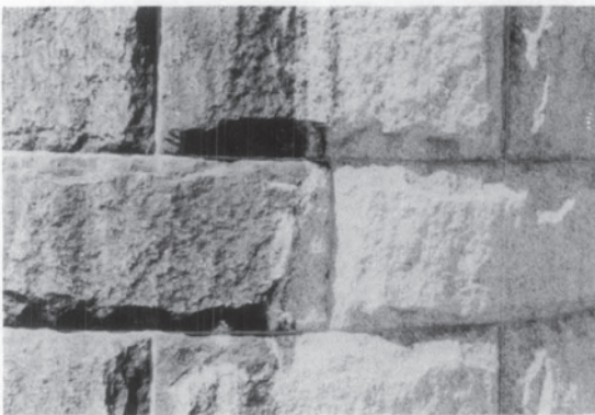
Chemical cleaning to remove urban dirt and pollution from granite without causing damage or abrasion to the surface of the stone.
