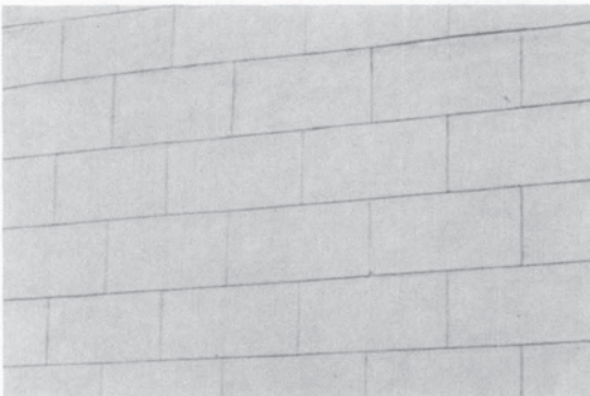
Stucco scored to resemble blocks of stone. Photograph: Anne E. Grimmer.
