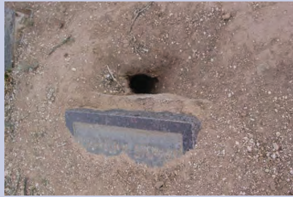
Figure C. Gophers and other burrowing animals produce uneven ground and holes that are trip and falling hazards to visitors and staff of historic cemeteries. Photo: Jason Church.
