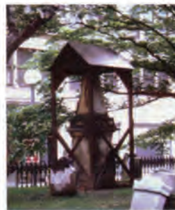
Fig. 4. Emergency stabilization by using an open-roofed shelter. Photograph by Frank Matero.
