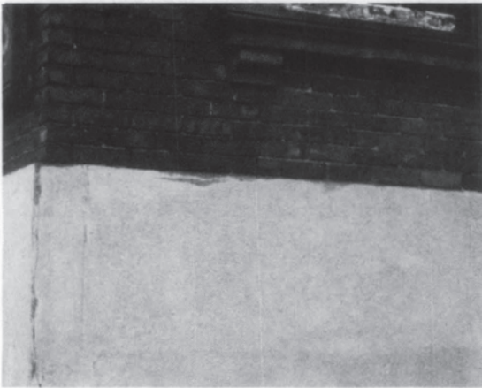
Parging over brick. Photograph: National Park Service.
