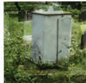
Fig. 5. Emergency stabilization using a closed, ventilated box around the structure. Photograph by Frank Matero.
