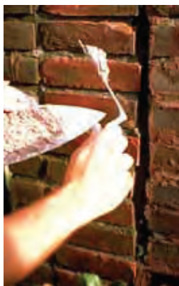
Soft mortar for repointing. Photo: John P. Speweik.
