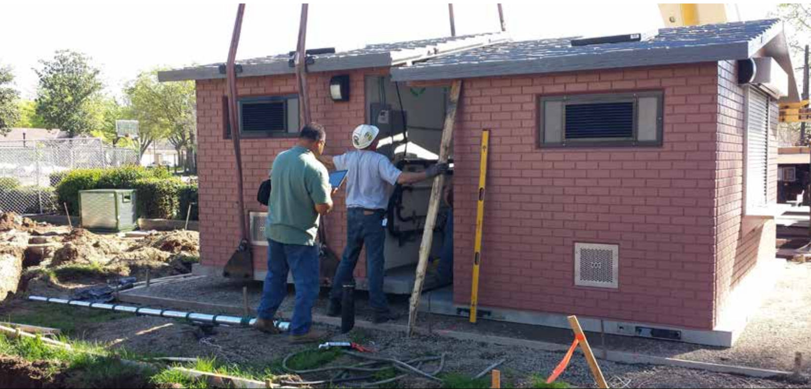
McClatchy Park restrooms undergo needed maintenance.
