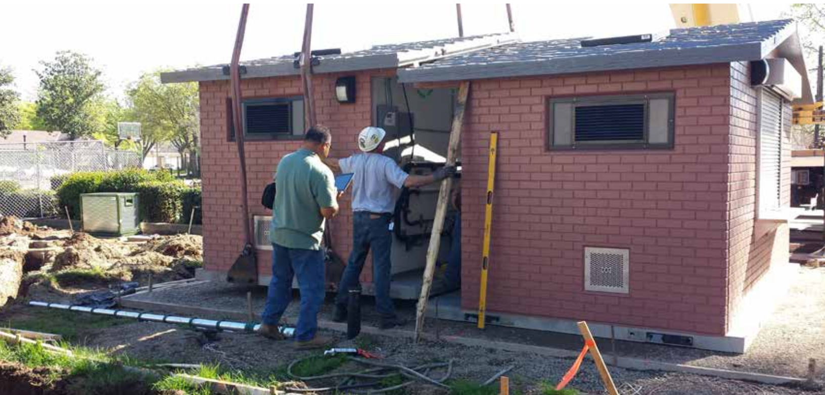
McClatchy Park restrooms undergo needed maintenance.
