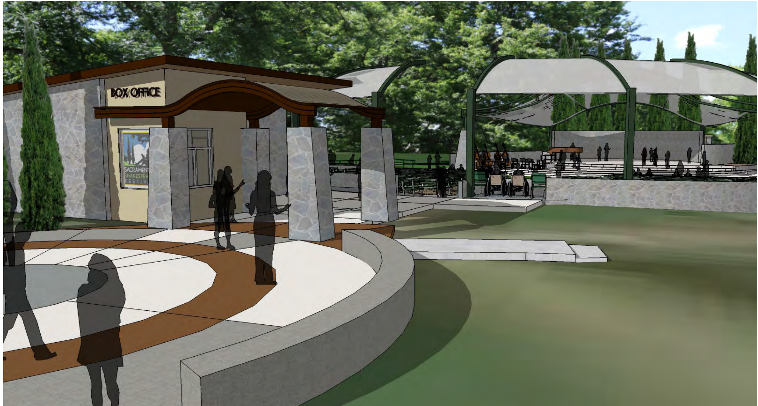
VIEW INTO ENTRY PORTAL ELEMENT
