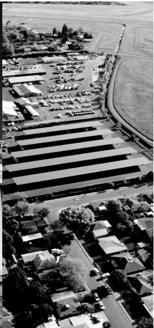
24th Street Solar Canopies
