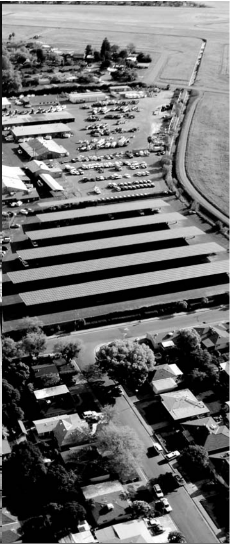
24th Street Solar Canopies
