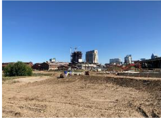
North View of the Railyards
