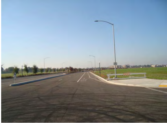
Viewing West on Delta Shores South Circle
