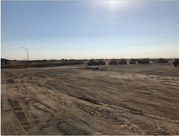
Overall View of Project
