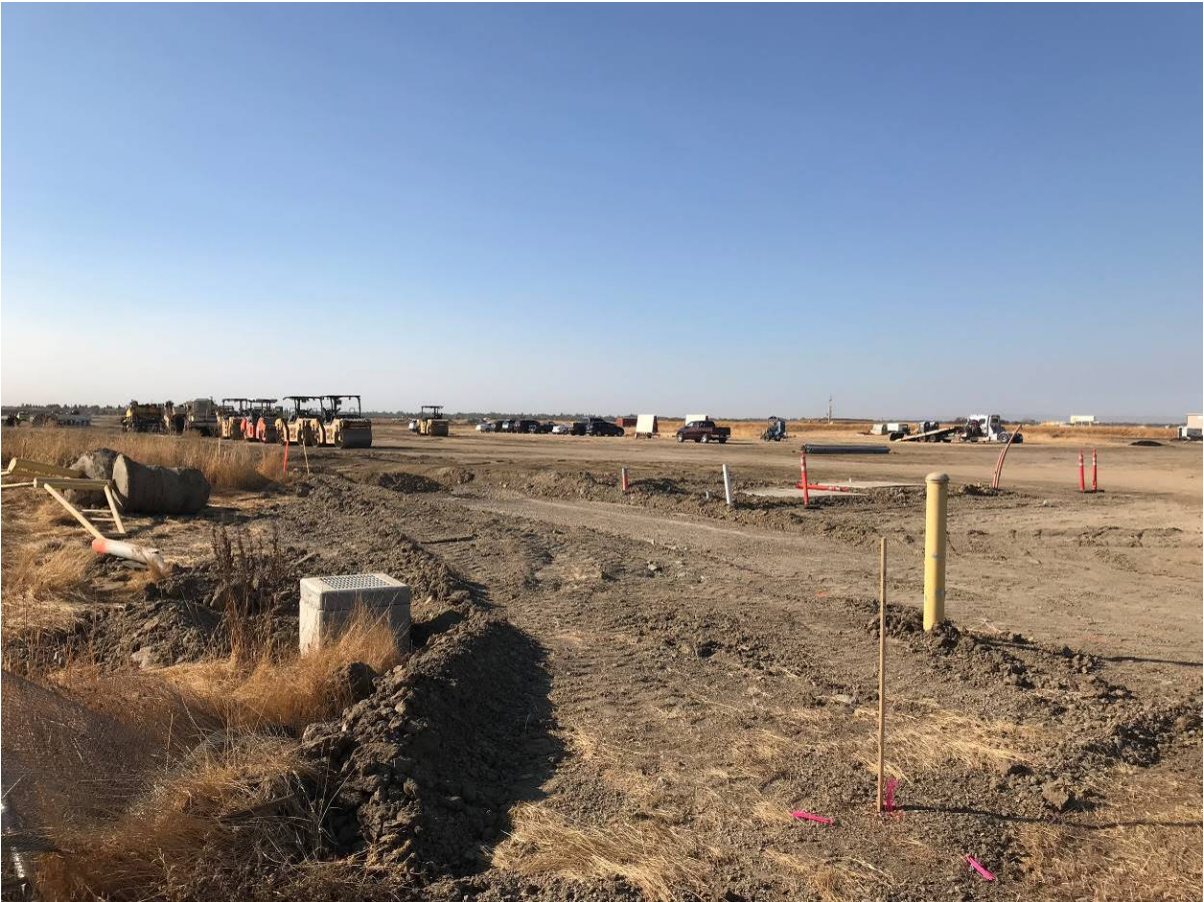
Overall View of Project
