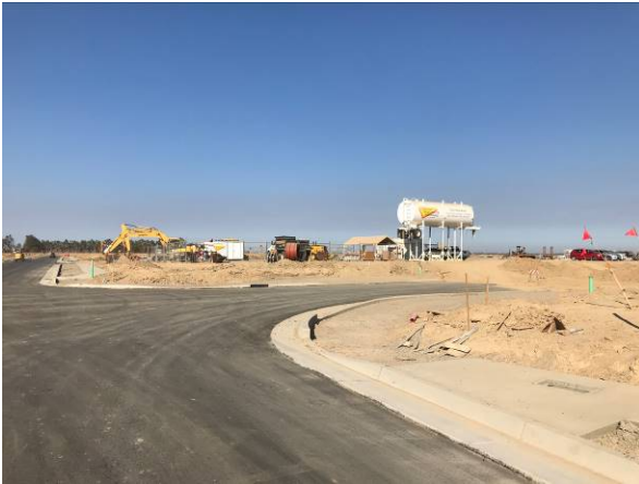
Site Improvement in Progress
