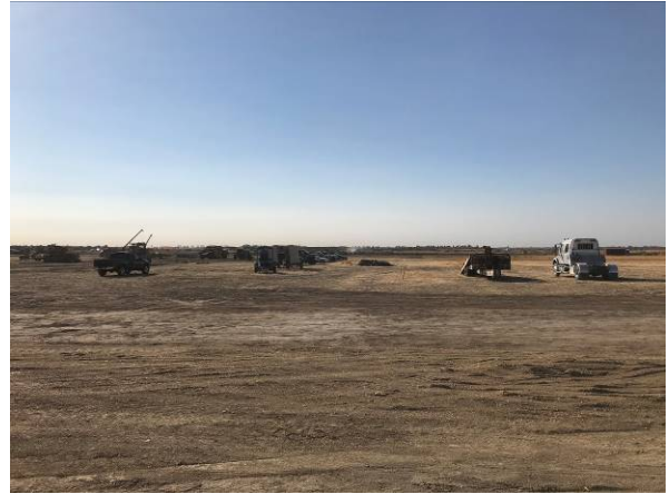
Overall View of Project
