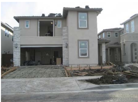
A partially completed home in Tax Zone 7
