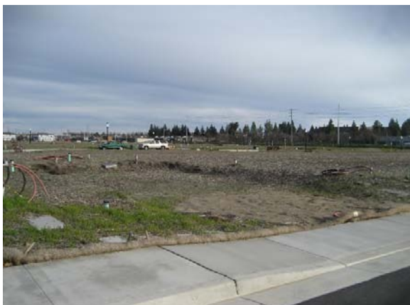
Looking southeast across Tax Zone 5, at an area where site work is complete but final map has not recorded
