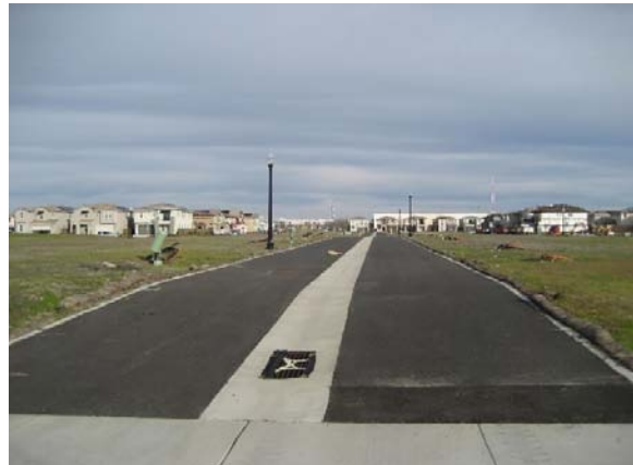
Completed alley drive within Tax Zone 6
