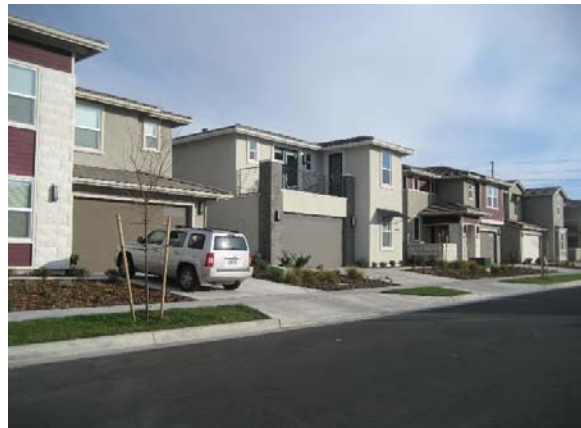
Completed/transferred homes within Tax Zone 7 (homes built by Anthem United)
