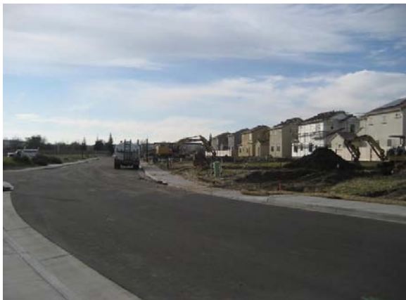
Looking west along Silver Almond Lane (Tax Zone 5)
