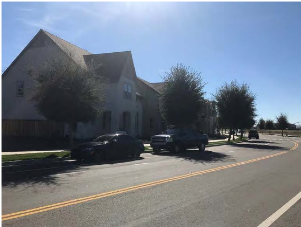
View of Finished Lots (Blackpine Curtis LLC) – Homes Under Construction
