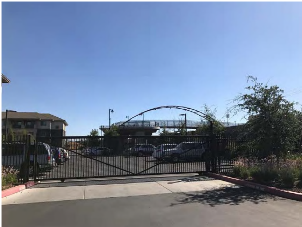
View of Pedestrian Bridge to Light Rail
