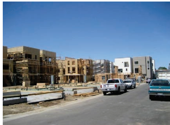
Looking north along City Flat Drive
