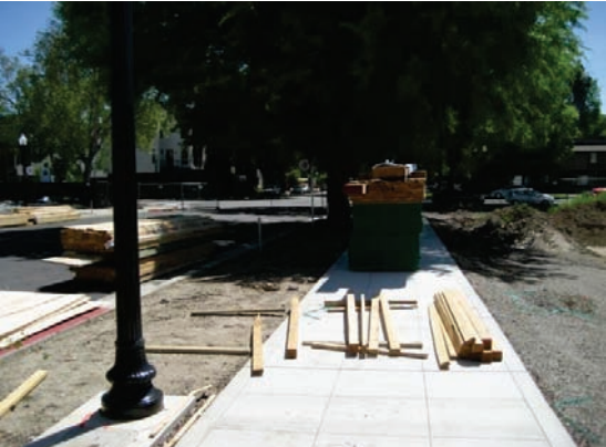
Looking south along 10 th Street
