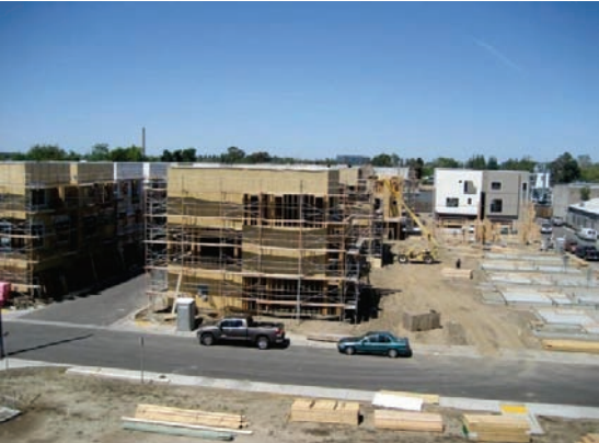
Looking north at the north block
