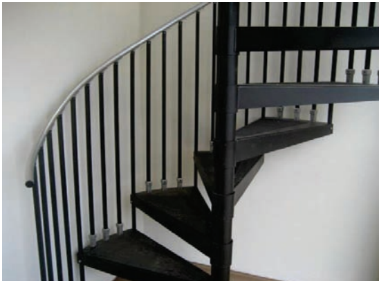
Circular staircase to rooftop patio
