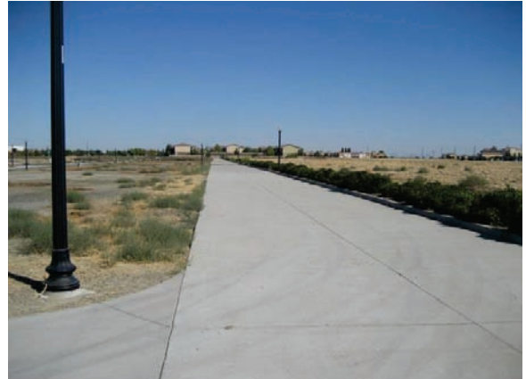
Finished alley drive within Village B (K. Hovnanian) (Photo Taken on September 18, 2016)
