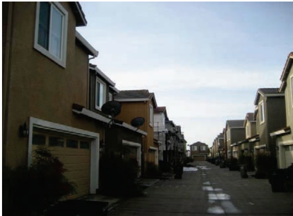
Alley drive at The Retreat by K. Hovnanian Homes (Photo Taken on)
