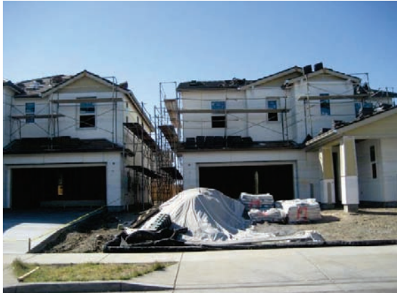
Homes under construction by Taylor Morrison Homes (Photo Taken on September 18, 2016)
