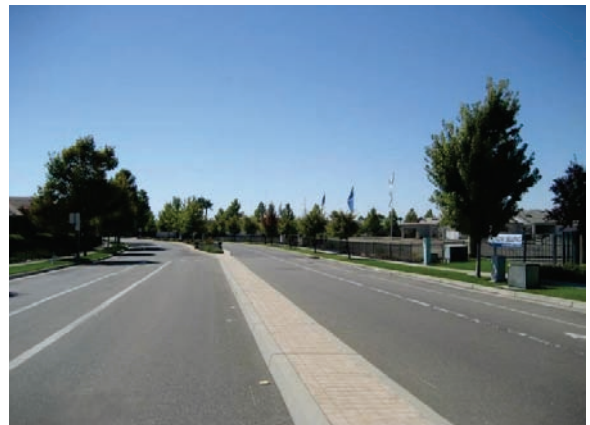
Looking south along Hovnanian Drive (Photo Taken on September 18, 2016)
