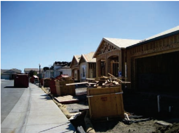
Homes under construction within Village G (Lennar) (Photo Taken on September 18, 2016)
