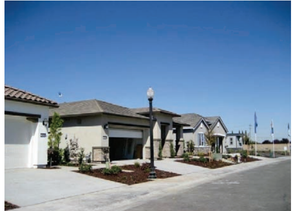
Models under construction by Lennar (Photo Taken on September 18, 2016)
