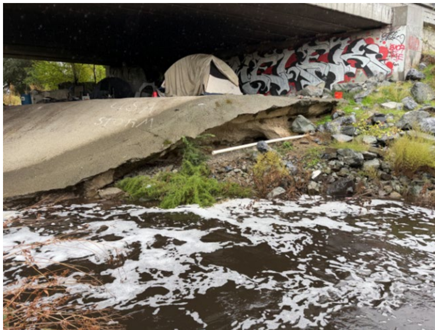
Figure 9. Roseville Road Bridge – Scour issues around Abutment 1
