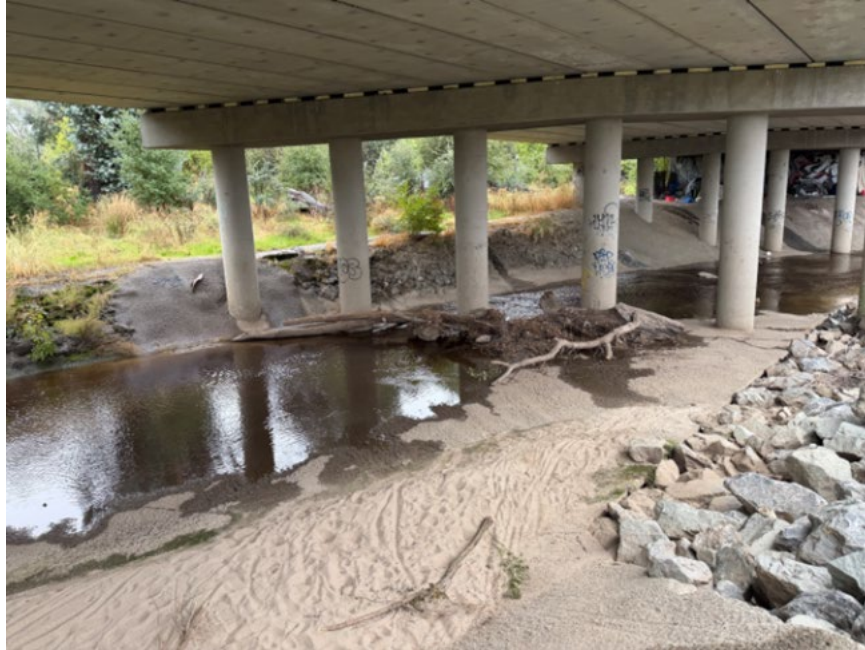
Figure 8. Roseville Road Bridge – Pier 3 with accumulated debris
