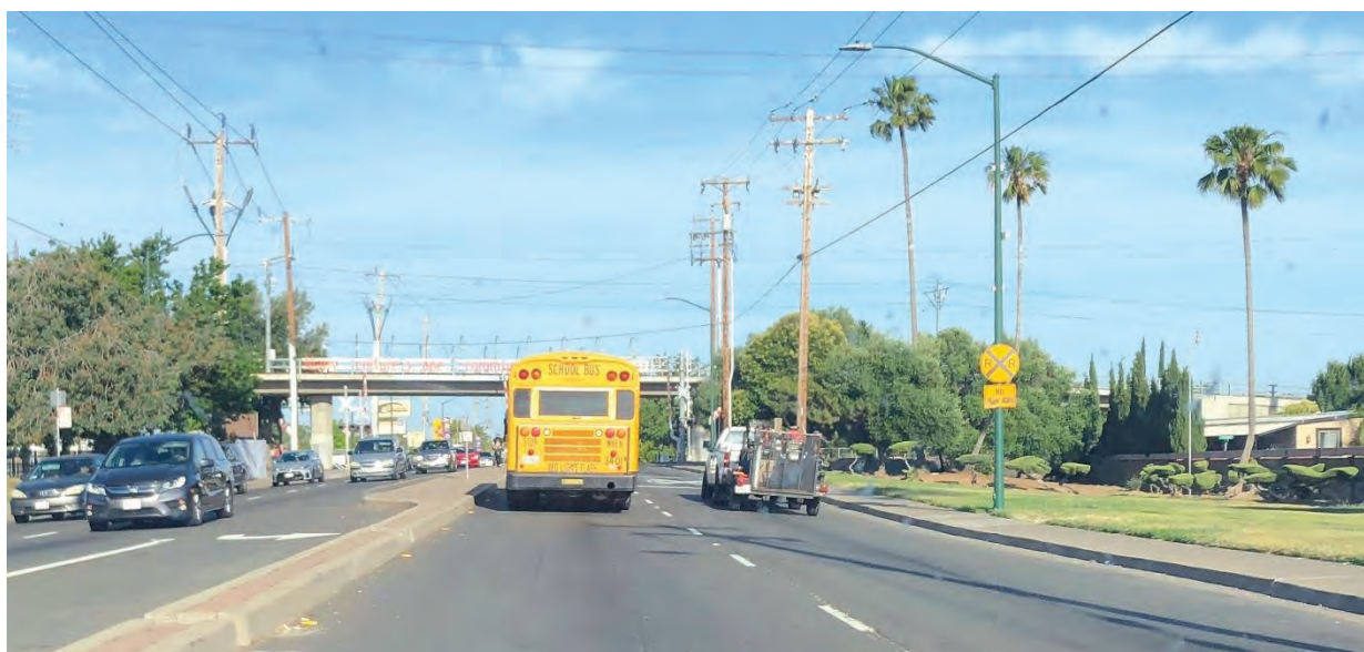
Figure 27: Florin Road and Light Rail Overcrossing
