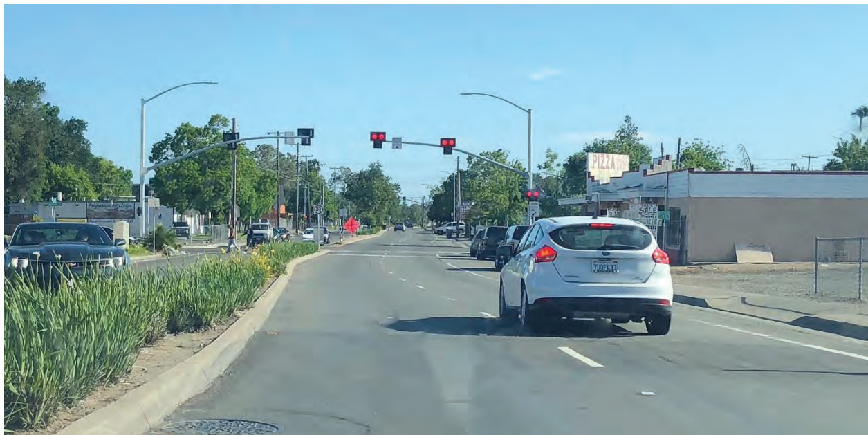
Figure 34: Marysville Boulevard/Roanoke Avenue HAWK
