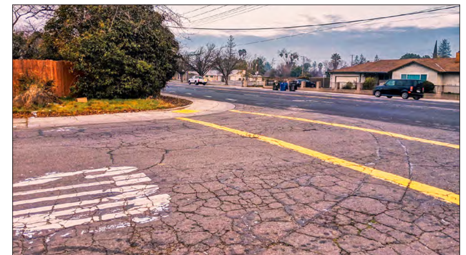
Northbound left turns at 19th Street and Meadowview Road can be challenging due to wall to the west blocking northbound sightline of oncoming eastbound traffic.
