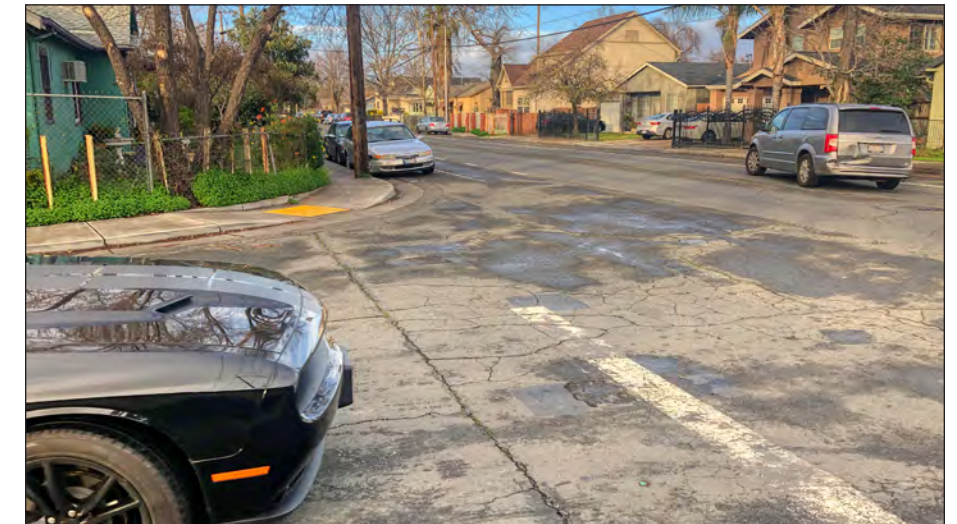
Parking on Martin Luther King Jr Boulevard obstructs sight lines for vehicles approaching from eastbound 26th Street.
