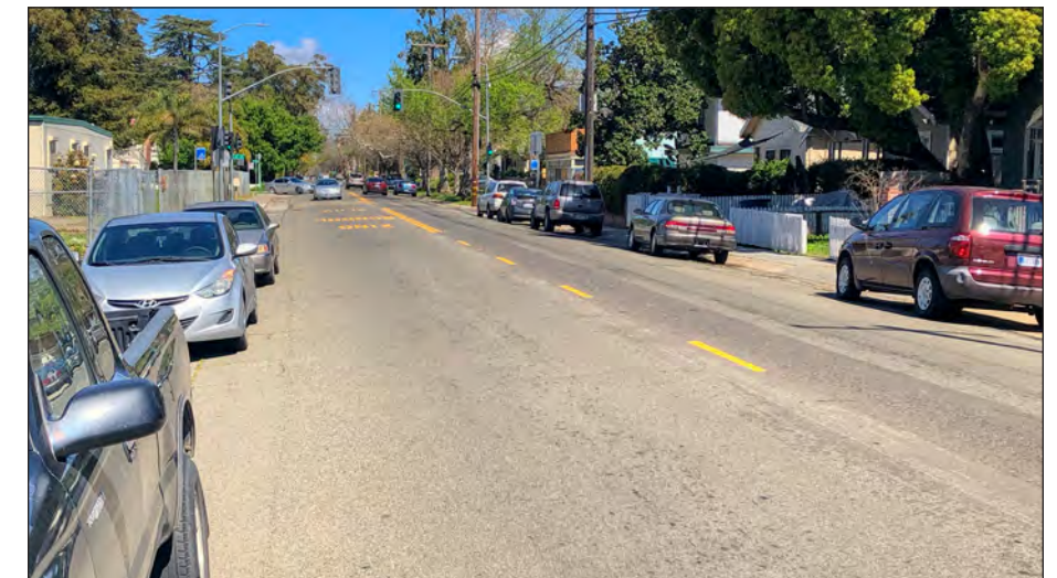
Franklin Boulevard runs adjacent to the school and is a highly trafficked and wide arterial street. School representatives perceive speeding along the street.
