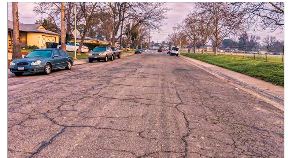
19th Street is a 36-foot wide roadway with on-street parking on both sides.
