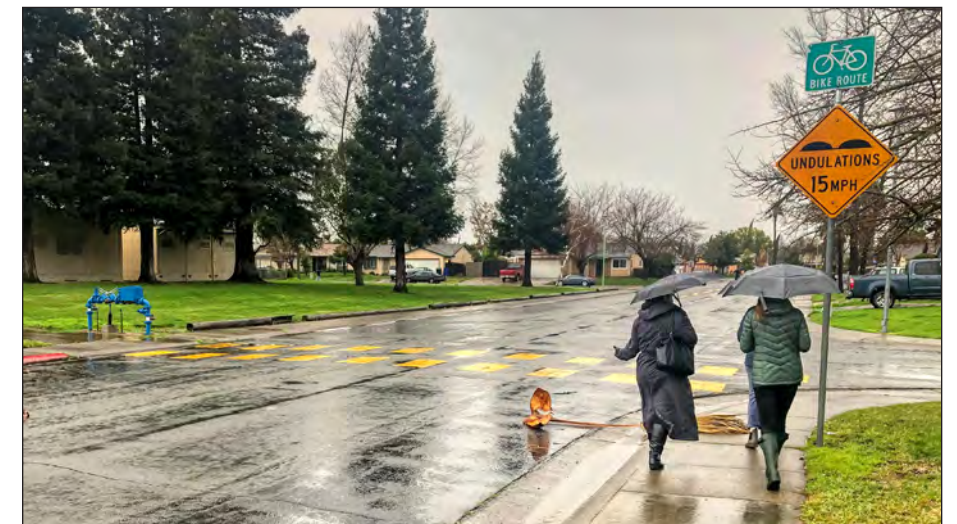
The uncontrolled crossing at Bamford Drive and Panos Court lacks school-area crosswalk signs and ADA-compliant curb ramps.
