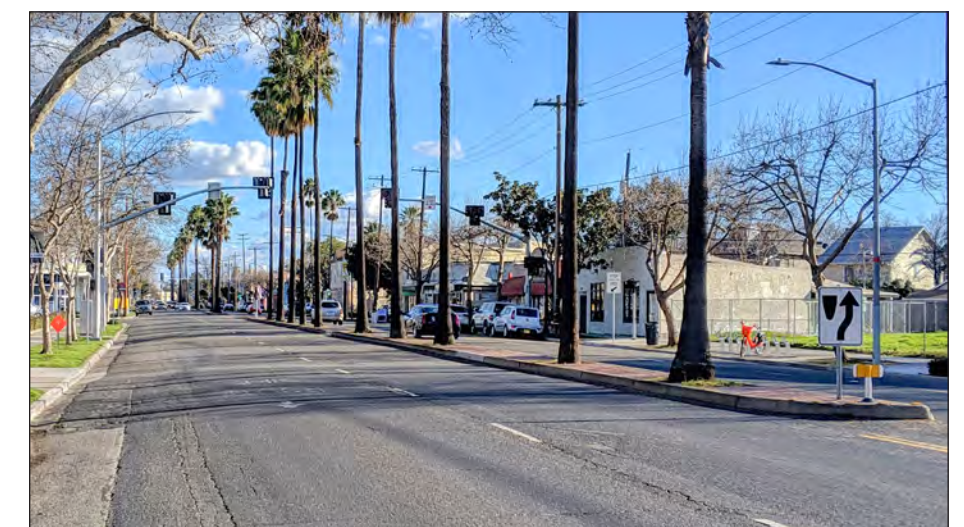
Broadway is a 65-foot wide arterial roadway. School administrators reported high speeds along Broadway
