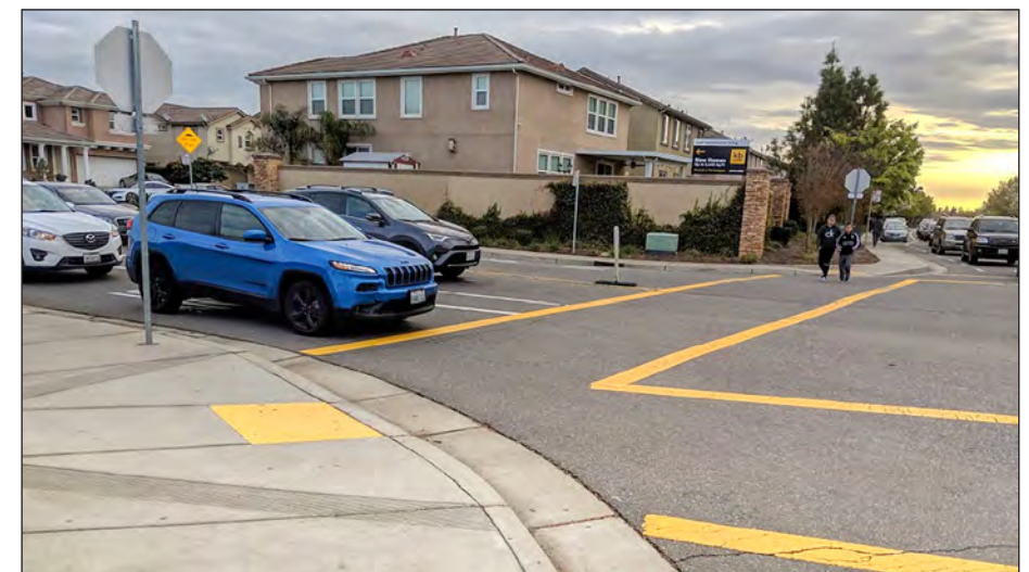
Multi-lane approaches at the all-way stop controlled intersection of North Park Road and Kokomo Drive results in confusion regarding which party has the right-of-way.
