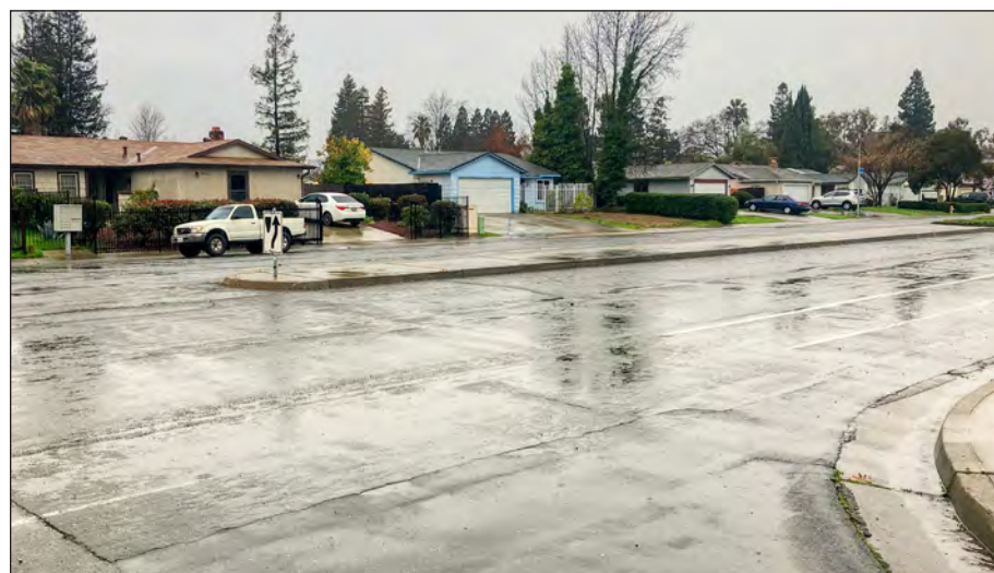
Bamford Drive at Center Parkway lacks a marked crosswalk across Center Parkway.
