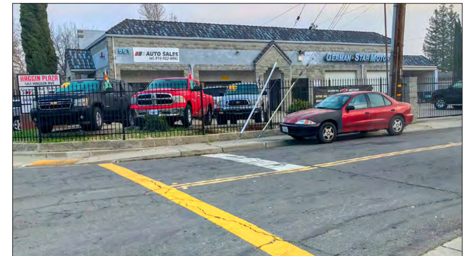
The Haggin Avenue / Northgate Boulevard intersection lacks red curb markings at the corners and vehicles have been reported parking adjacent to the curb ramps.
