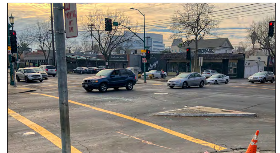
There is a raised triangular island at the Alhambra Boulevard and J Street intersection. Some motorists roll through the right turn at this approach, as well as causes a hindrance for bicycles.
