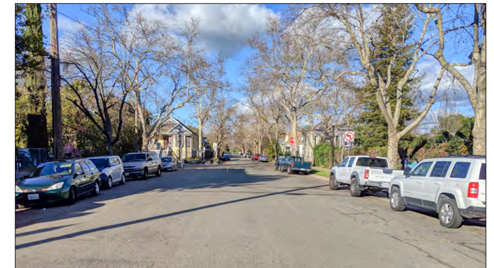
33rd Street is a 45-foot wide roadway with on-street parking on both sides.
