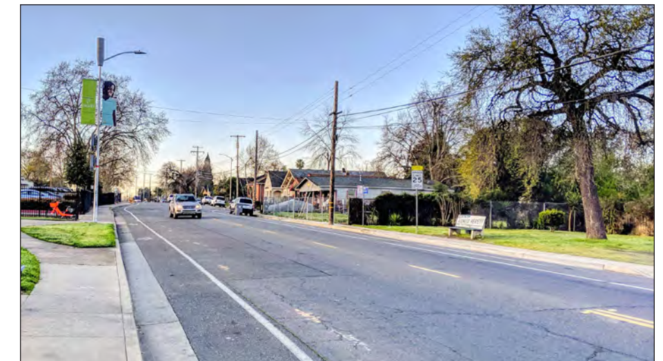
The northbound vehicle lanes in front of the school are between 16 and 20 feet wide.
