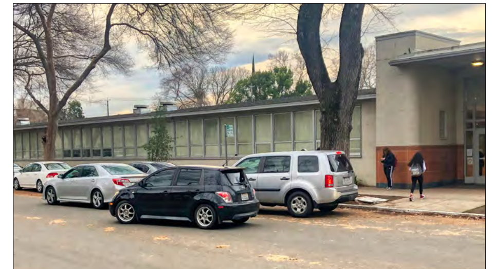
Vehicles double park on V Street due to insufficient loading zone length.
