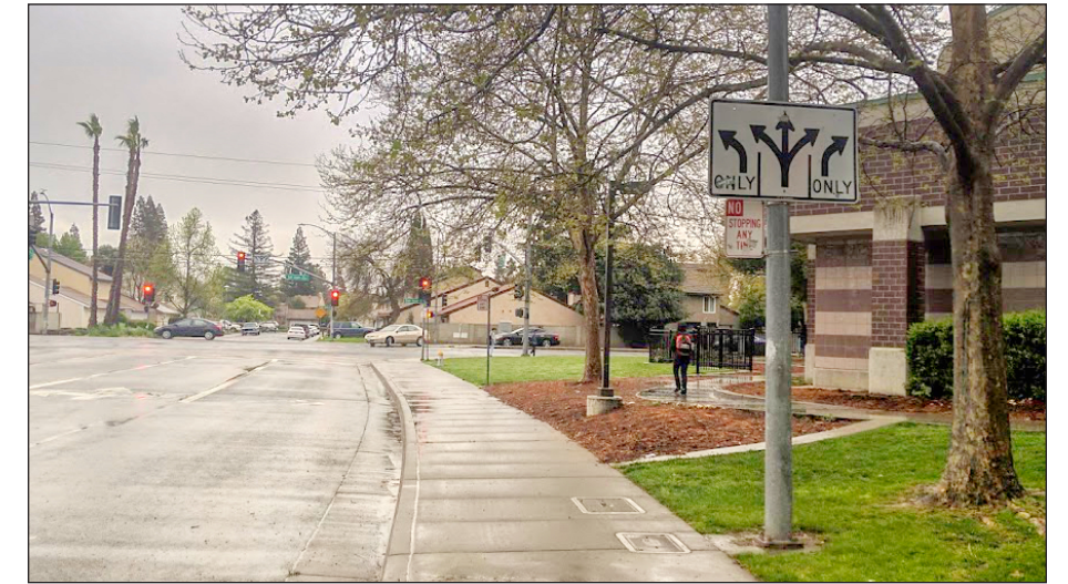
The configuration of the Fong Ranch Road and San Juan Road intersection has two right-turn lanes, which can result in potential conflict with pedestrians crossing the western and northern crosswalks.
