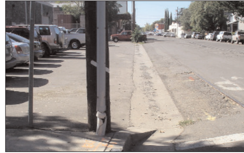
Vee gutters maintain the shared roadway concept on R Street.
