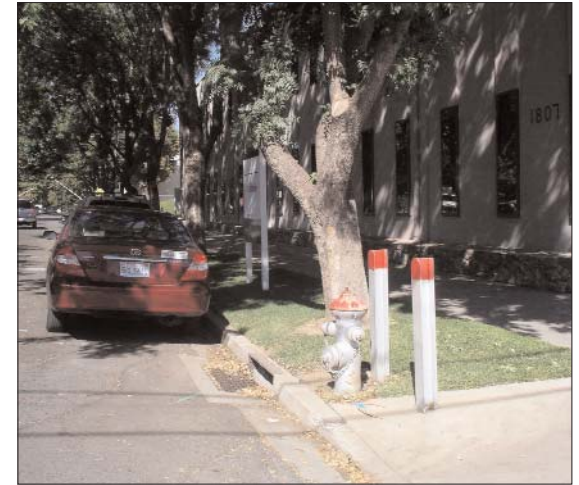
Hydrant and sewer system
