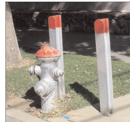
Bollards will be used to protect fire hydrants along the street.
