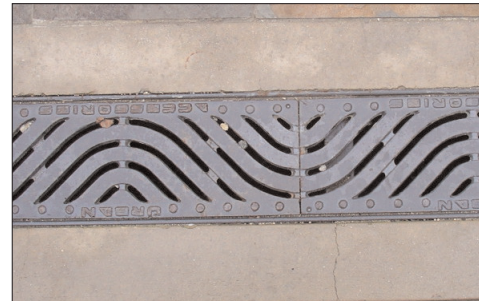
A slotted drain system would respect the inique industrial character of R Street's history.
