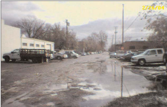
Flooding on R Street
