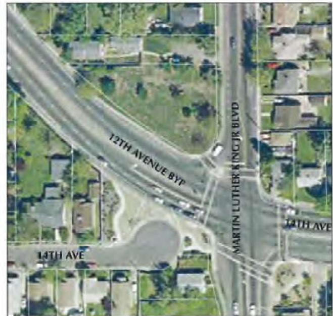
Existing aerial view
