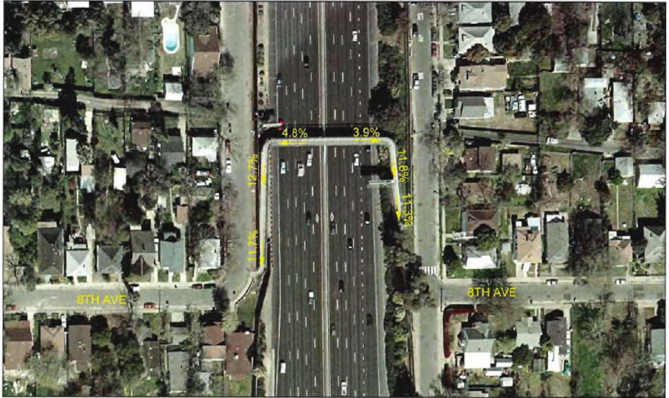
PEDESTRIAN BRIDGE OVER STATE ROUTE 99 AT 8TH AVE NORTH OF 12TH AVE INTERCHANGE
