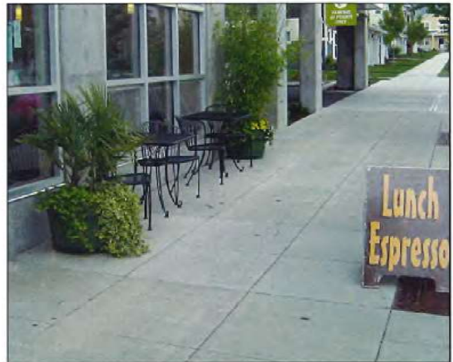
Scored concrete sidewalks
