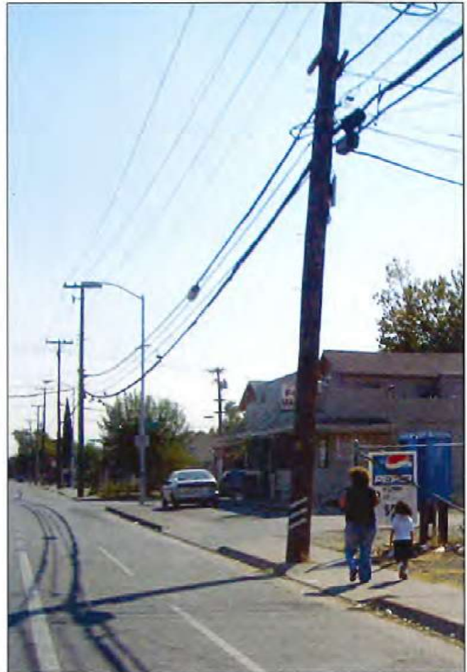
Overhead utilities create sidewalk obstructions and are unsightly
