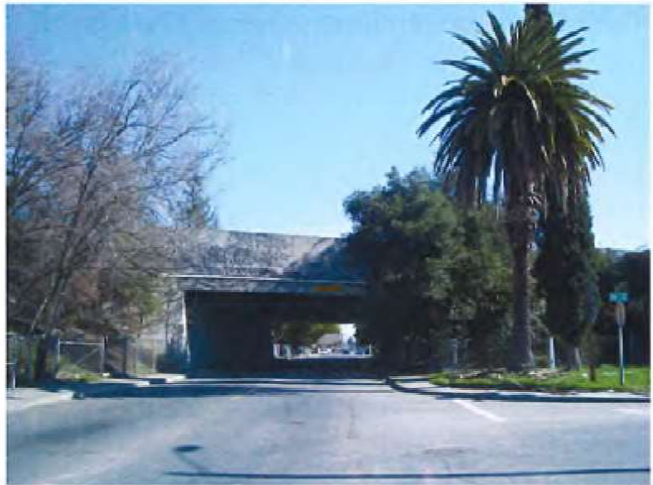
Existing tunnel looking east
