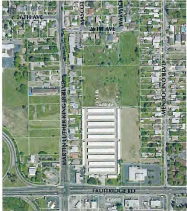
Existing aerial view
