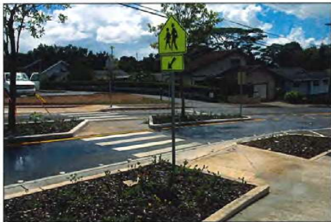
Photo of pedestrian oasis with staggered pedestrian approach.
