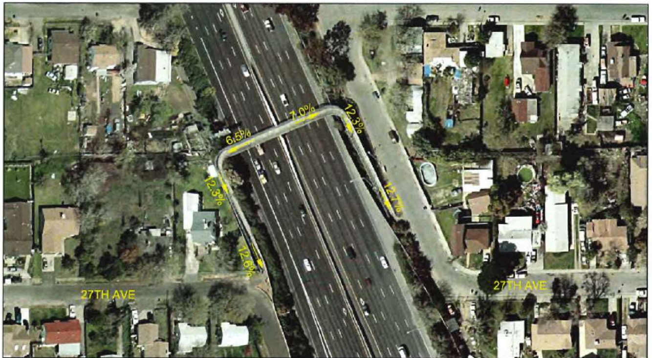
PEDESTRIAN BRIDGE OVER STATE ROUTE 99 AT 27TH AVE NORTH OF FRUITRIDGE INTERCHANGE
