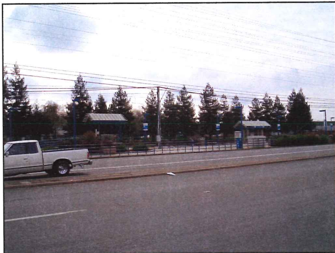
College Green LRT Station
