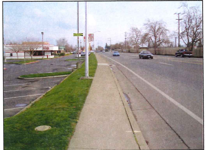
Existing Sidewalk at Raley's Shopping Center
