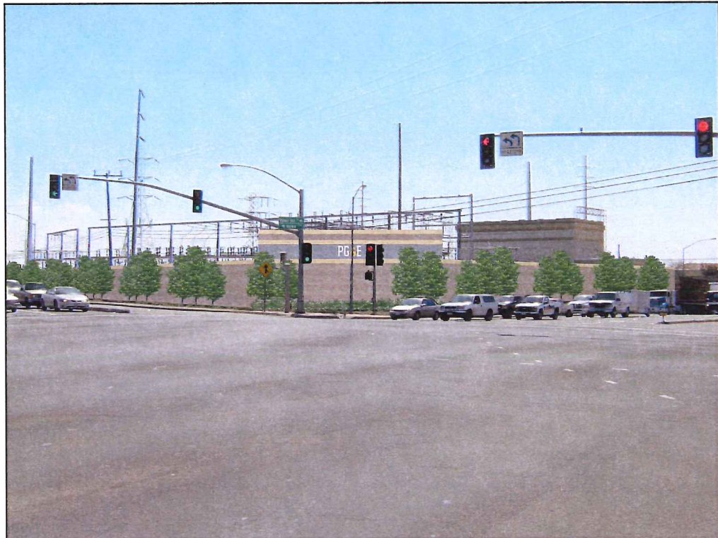
PG&E Substation Screen Wall
