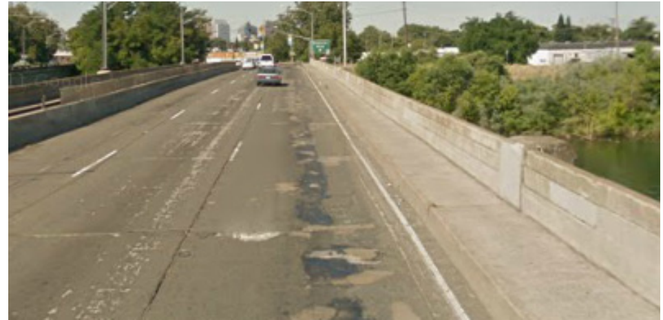
Existing Narrow Sidewalk on SR- 160 (looking towards downtown)
