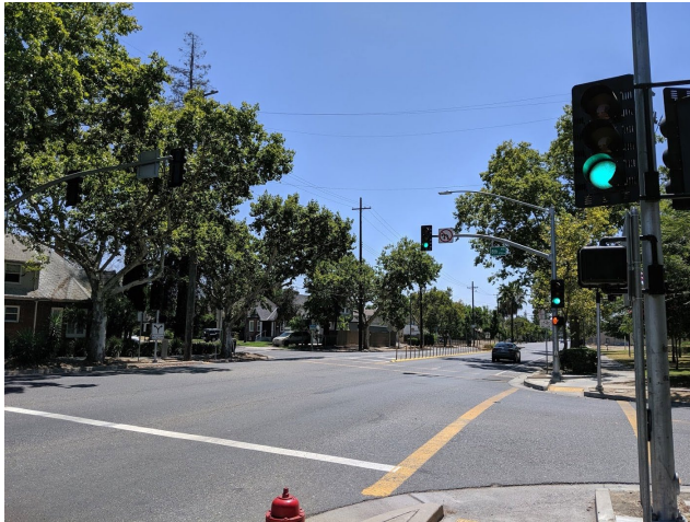
Typical signalized intersection
