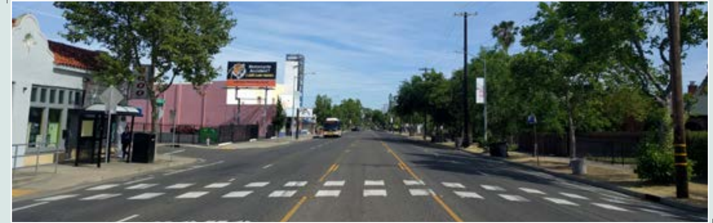
This crosswalk at 11th Avenue serves bus stops and needs signalization to improve safety
