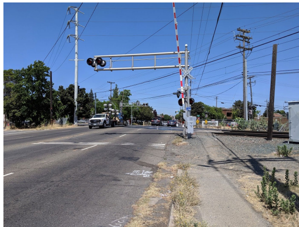
34 th Street light rail crossing facing north
