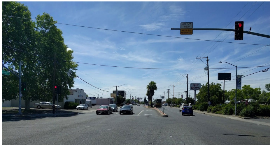
Existing street section with raised median on approach to intersection
