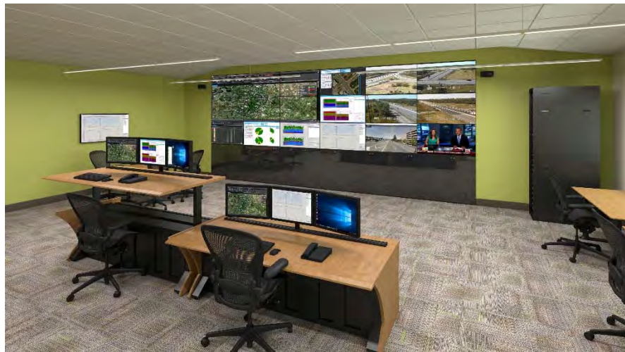
Typical Traffic Operations Center (TOC) rendering showing Workstations and a Video Wall
