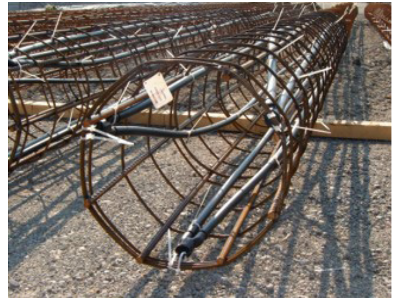
Figure 7.6 Ground Loop Tubing within Rebar Cages of Structural Piles
