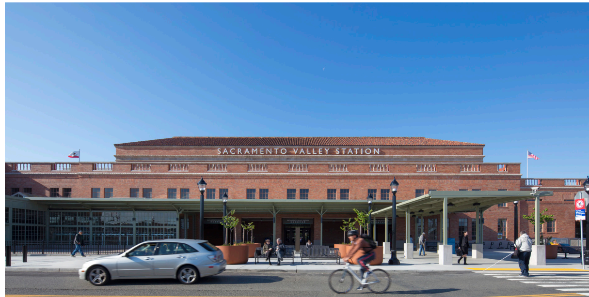
Existing Sacramento Valley Station north entrance
