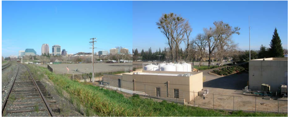
The existing reservoir (seen at right of photo) may be relocated or capped at the level of the adjacent levee.
