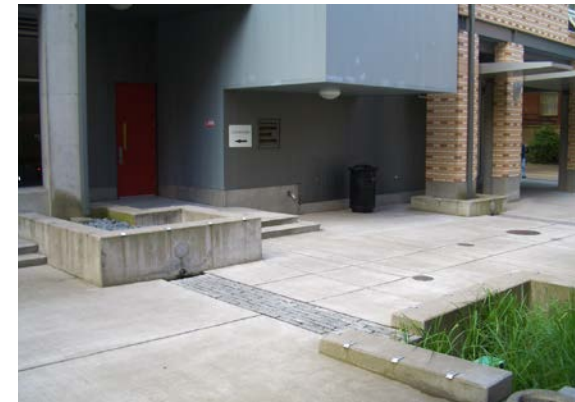
Rain garden detail - Portland, OR
