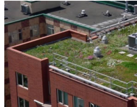
Green roofs aid in stormwater management and energy efficiency.
