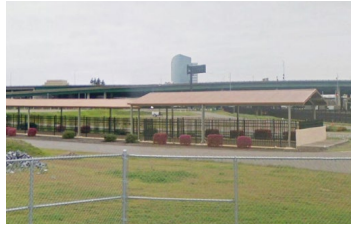
Existing Canopy structures
