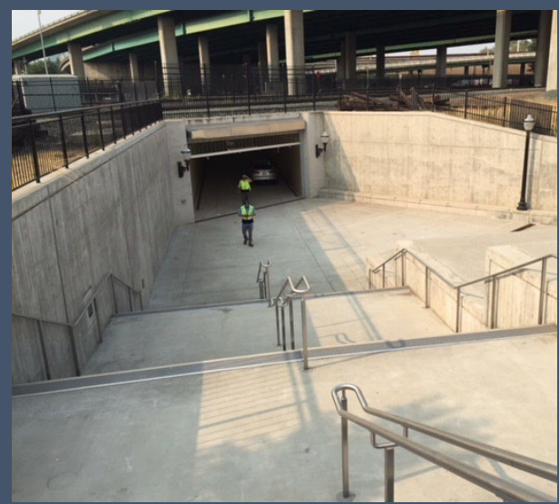
North of Tracks Stair and Ramp
