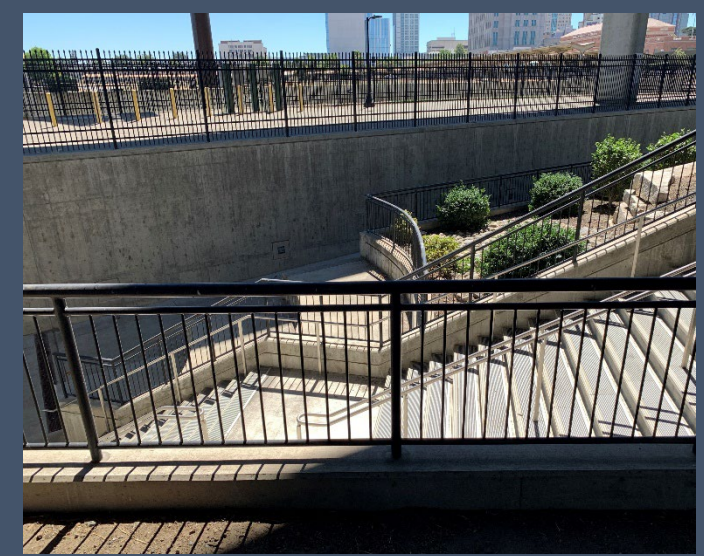
South of Tracks Stairs and Vehicle Ramp
