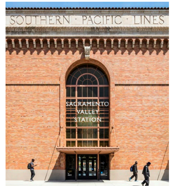
Sacramento Valley Station at the end of Phase 2, Year 2017. Image credit: Tim Griffith Photography.
