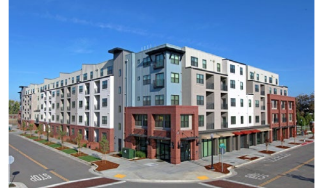
Cannery Place. Image credit: Kuchman Architects PC
