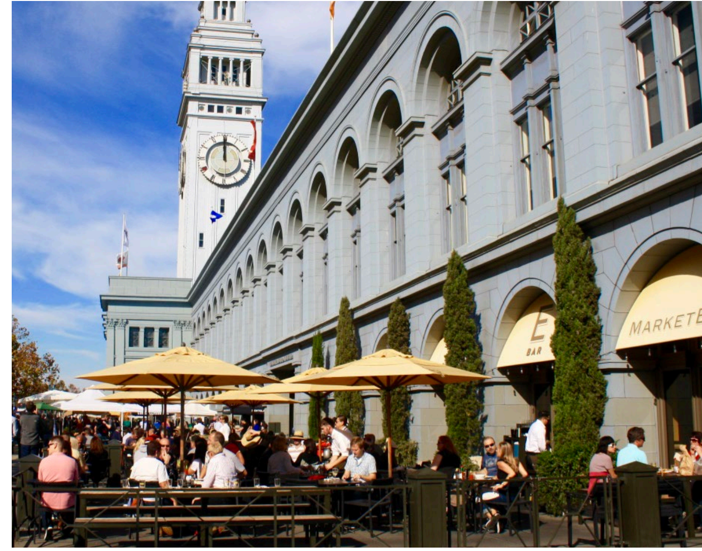
Ferry Building, San Francisco, CA
