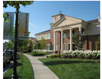
This new building at Kokomo Drive welcomes the pedestrian.
