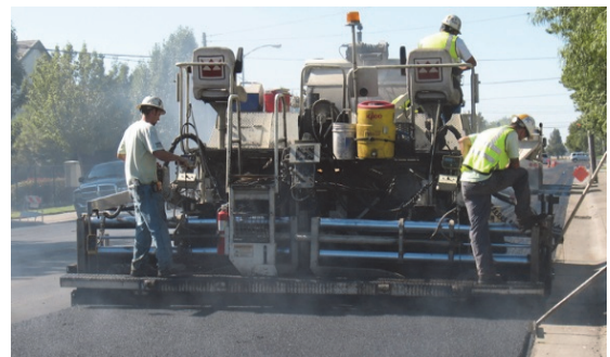
Street overlay in progress
