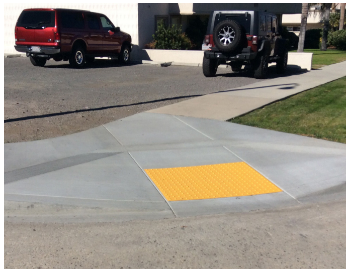
Figure 11. Example Curb Ramps
