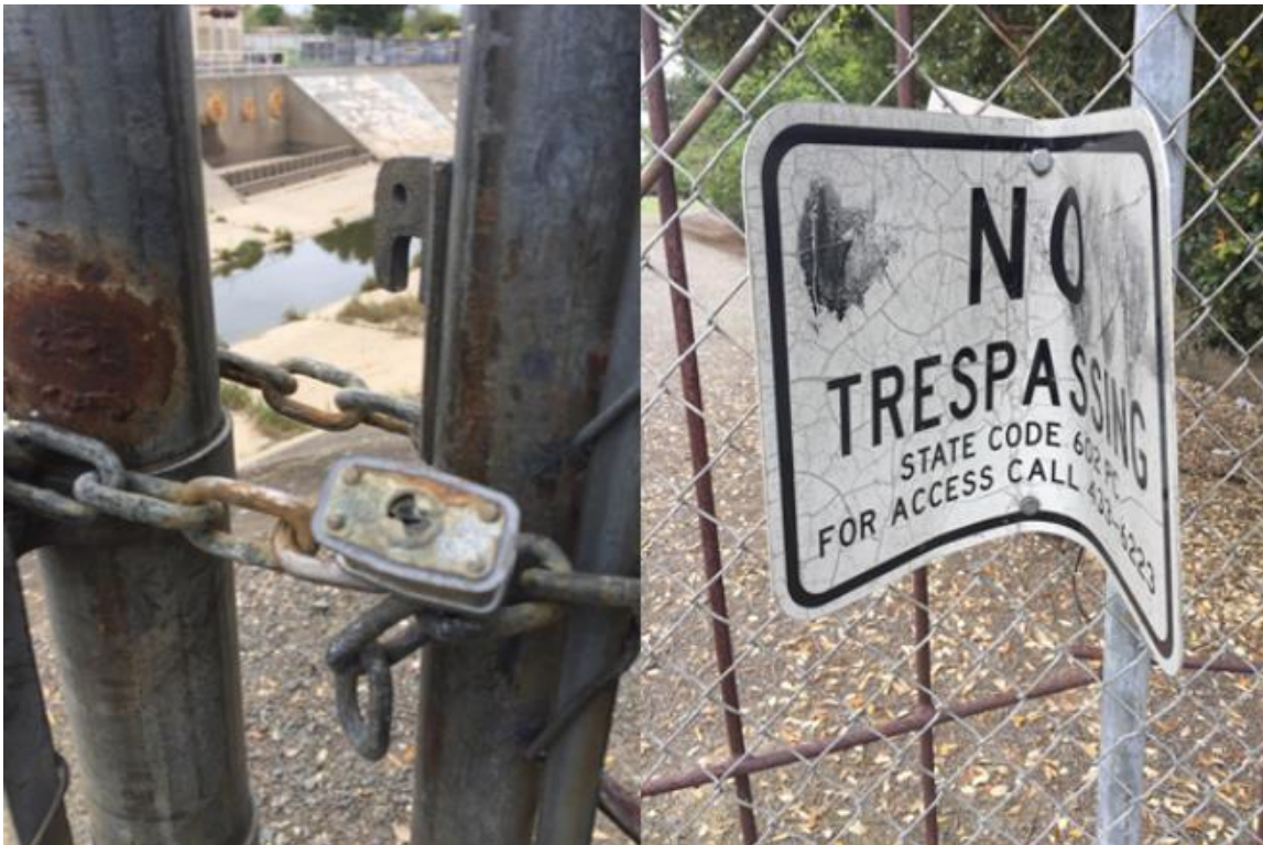
Figure 2. City locks and gates located at Logan St. prevent community members from actively using the creek corridor.
