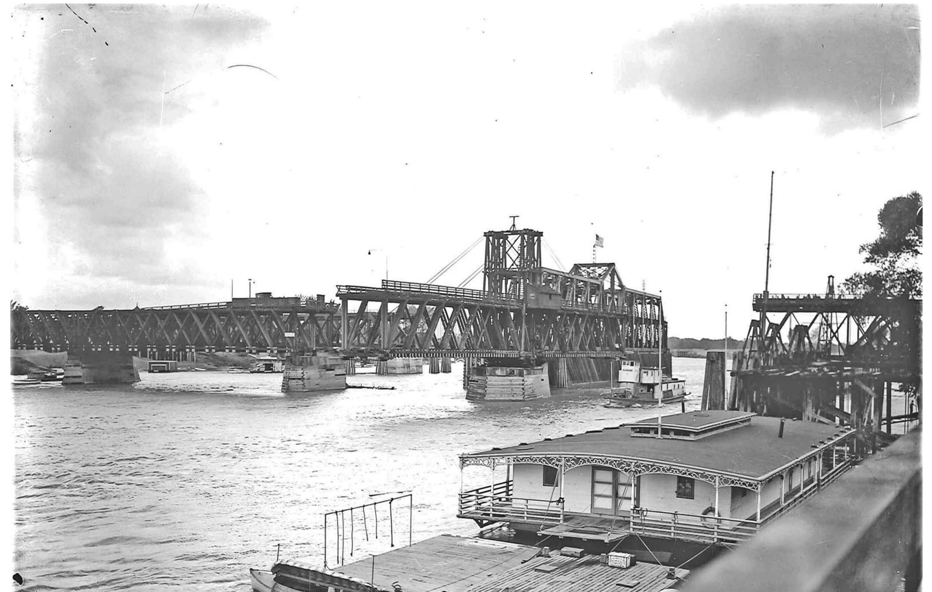
Southern Pacific Bridge and I Street Bridge Bridges open
