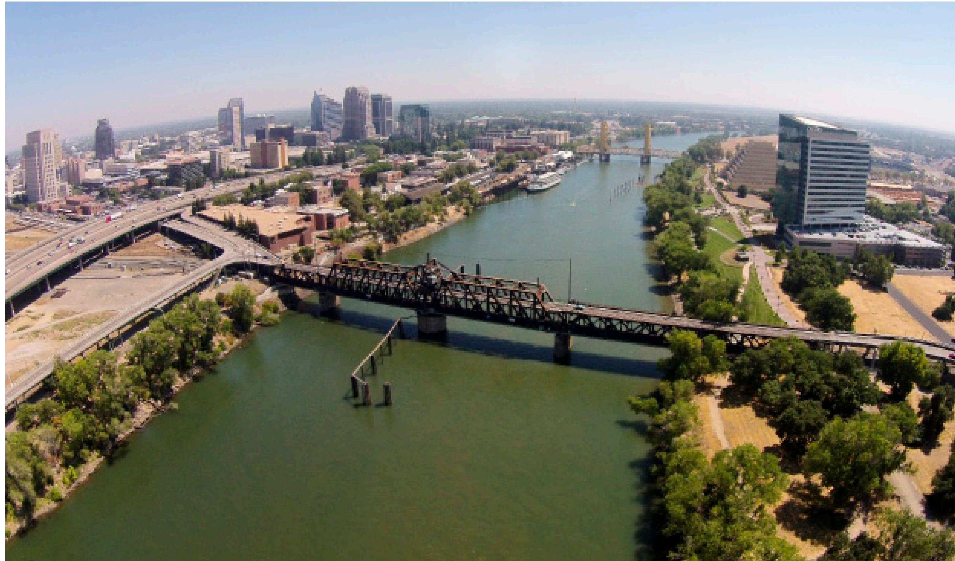
The existing I Street Bridge with viaducts
