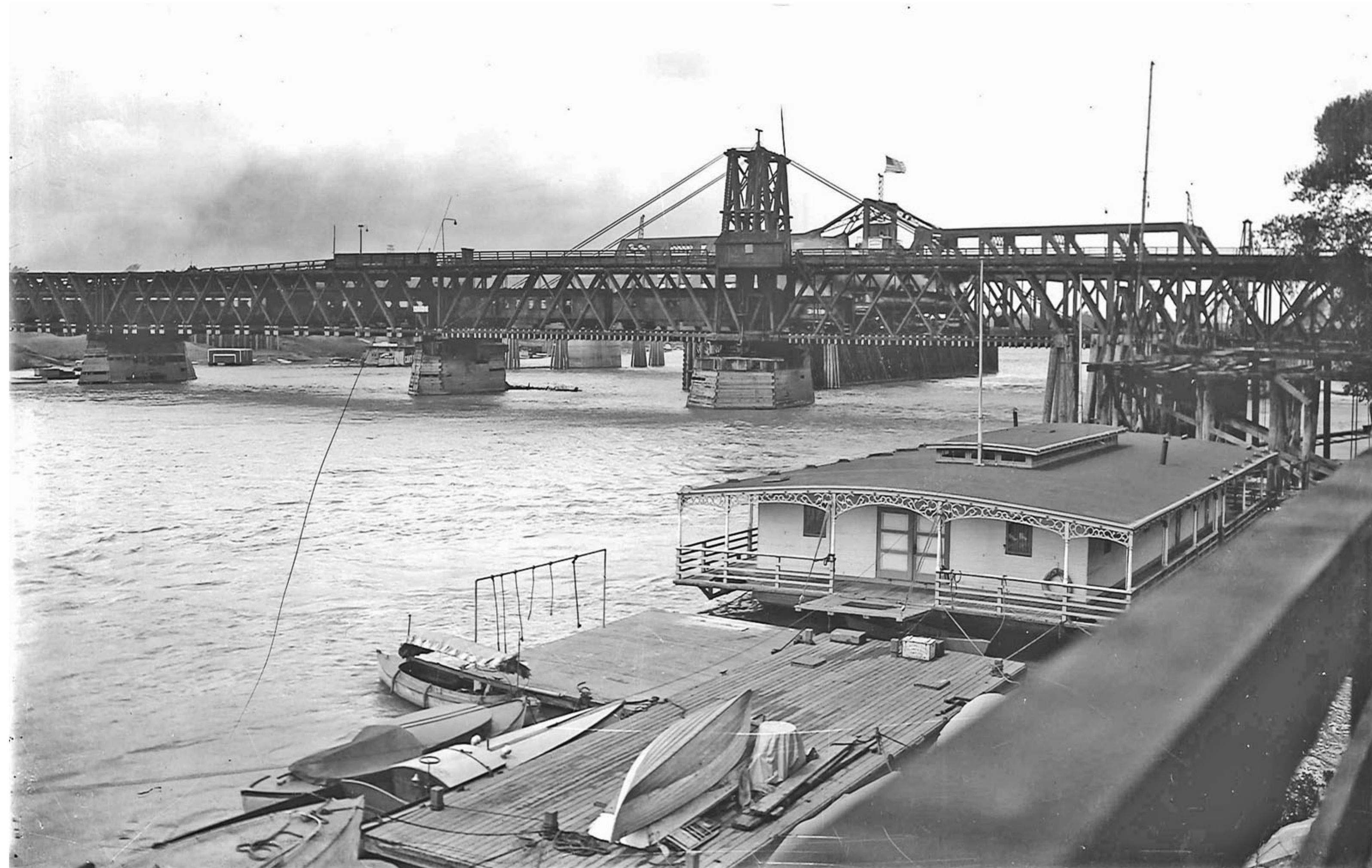
Southern Pacific Bridge and I Street Bridge Bridges closed; train crossing
