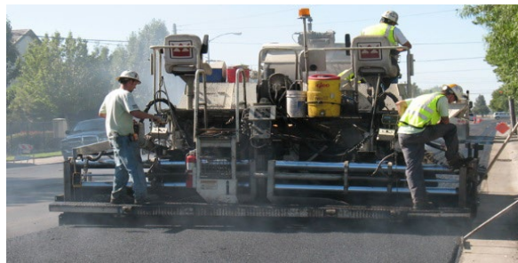
Street overlay in progress
