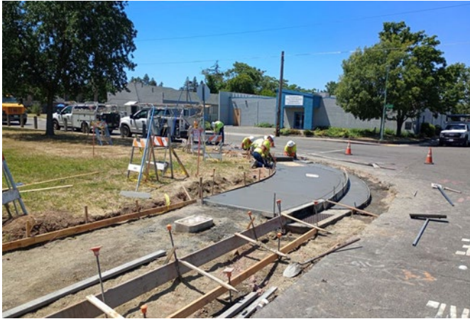
Grand Ave sidewalk gap closure construction
