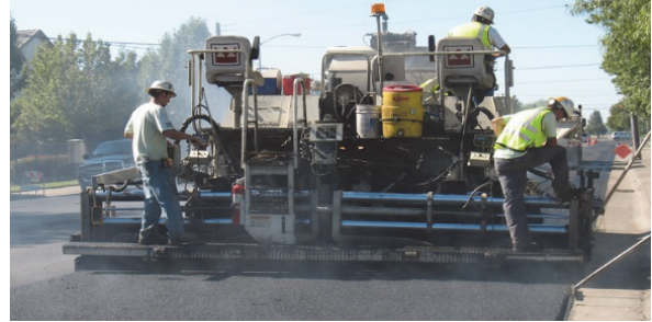
Street overlay in progress
