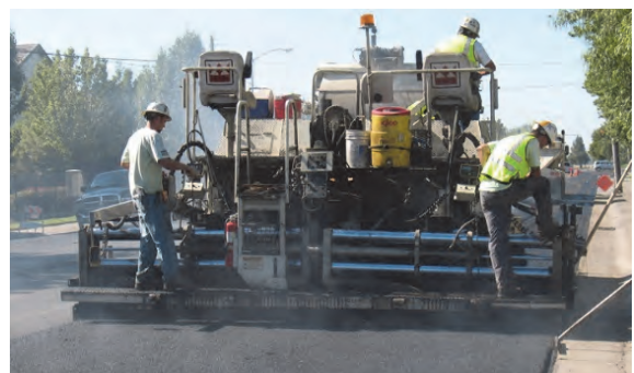
Street overlay in progress
