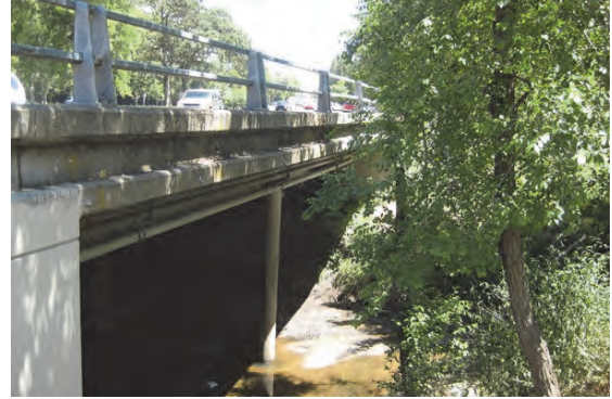
Auburn Boulevard Bridge at Arcade Creek (looking northeast)
