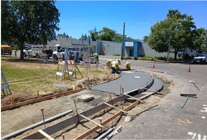
Grand Ave sidewalk gap closure construction
