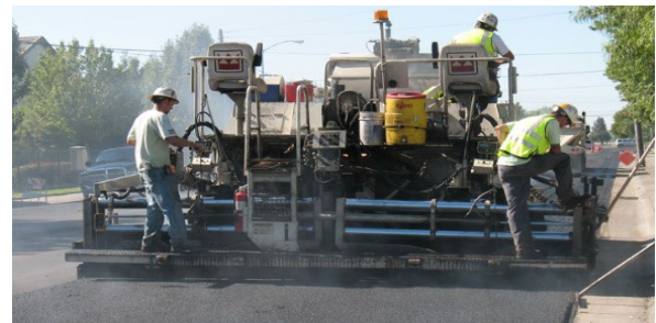
Street overlay in progress
