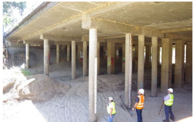
Inspection of Watt Ave Bridge at Arcade Creek
