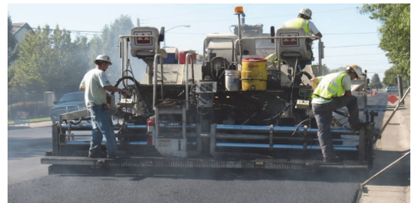
Street overlay in progress
