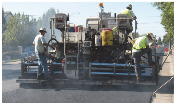
Street overlay in progress
