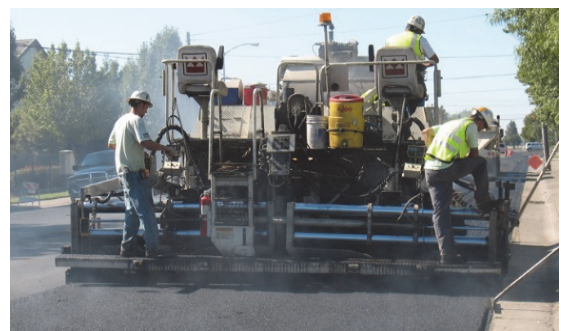
Street overlay in progress
