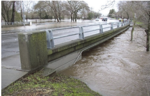
Auburn Boulevard Bridge during flood event
