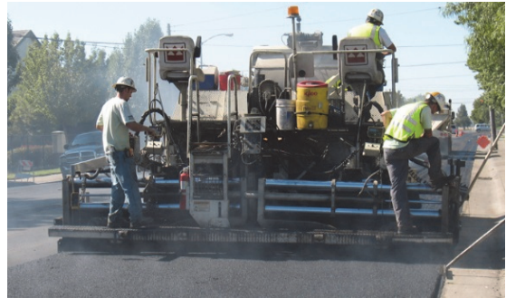
Street overlay in progress
