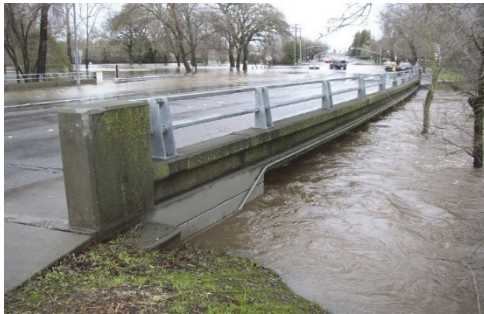
Auburn Boulevard Bridge during flood event
