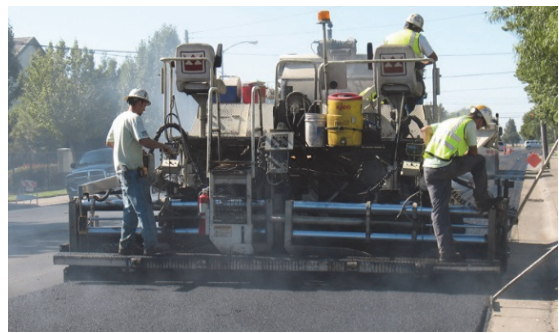
Street overlay in progress
