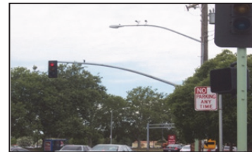
Traffic Signal Safety Program
