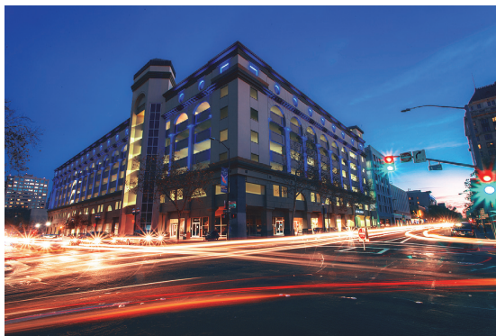
Renovated City Hall Garage
