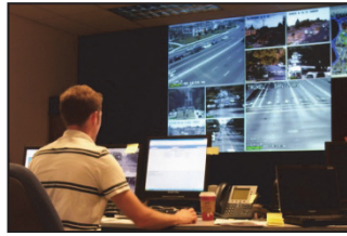
Traffic Operations Center
