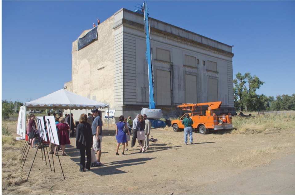
Site of the future Powerhouse Science Center
