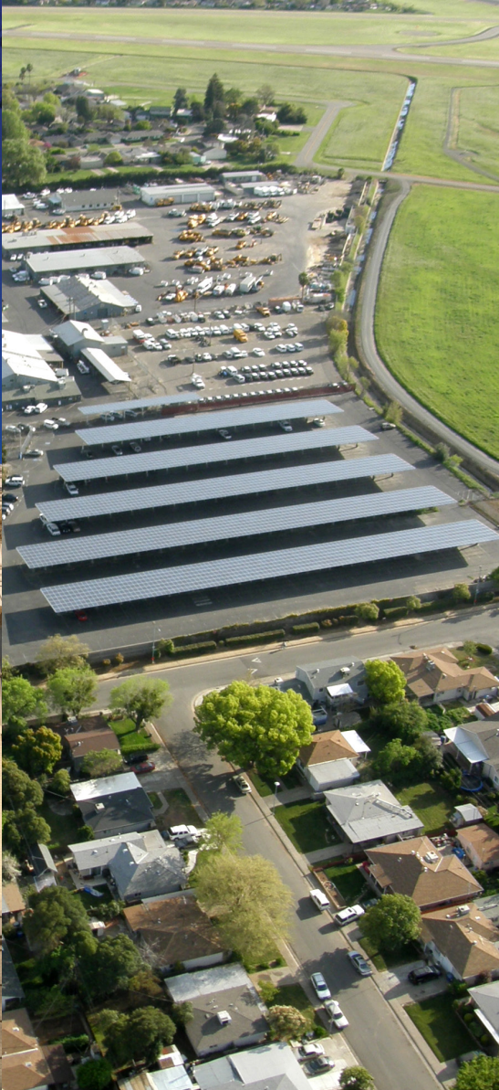
24th Street Solar Canopies
