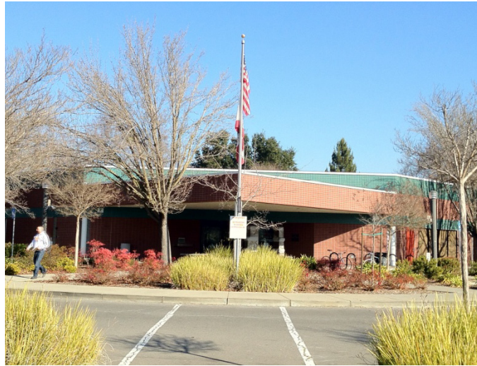
Belle Coolegge Community Center Deferred Maintenance Project
