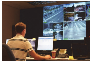
Traffic Operations Center
