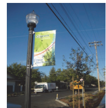
Neighborhood Street Light Replacement
