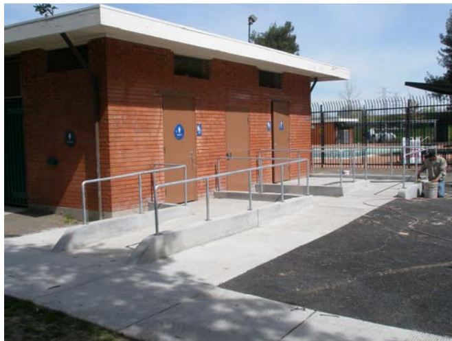
ADA Restrooms at Glenn Hall Park
