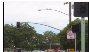
Traffic Signal Safety Program
