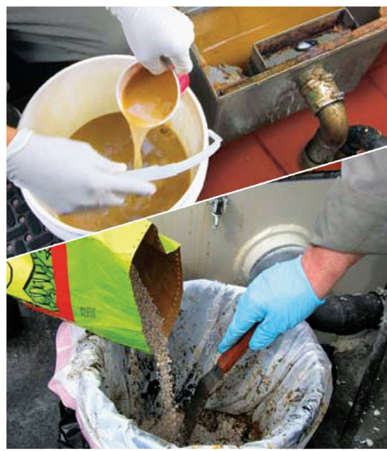
Keep grease traps and interceptors clean.
