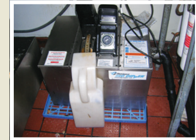
Sample Indoor Automatic Grease Trap
