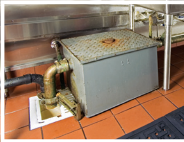
Sample Indoor Manual Grease Trap
